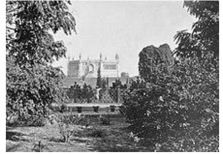
The Bibighar Well site where a memorial had been built by 1859. Samuel Bourne , 1860.
